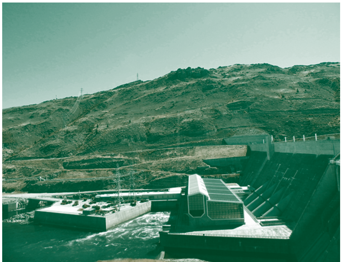
The Clyde River dam in summer – store or run? 14
